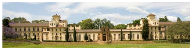
Physics building during construction 1923-1925 and Physics building today. Photograph provided by Tim Bedding.
