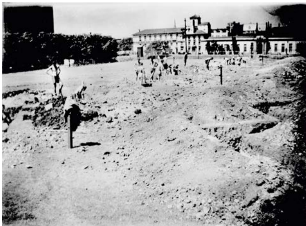
Air raid trenches being dug in front of the Physics building. 1940s. REF-00050156
